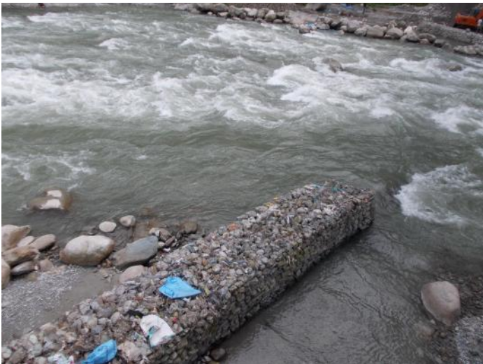
Spurs wall on Sikkim side
