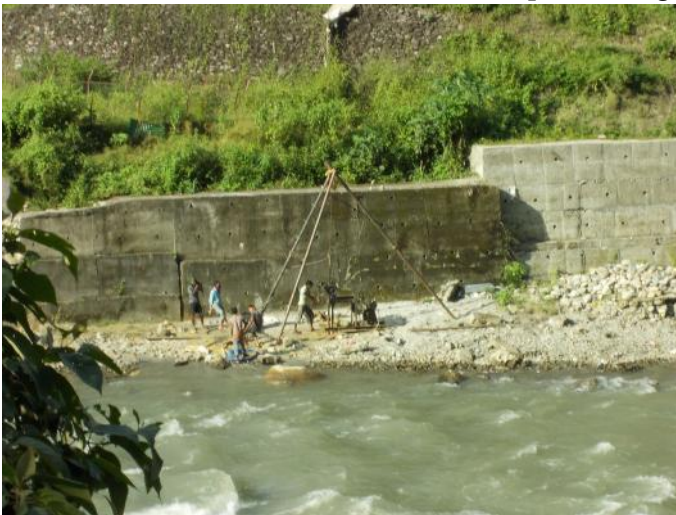
Geotechnical Investigation at bridge site
