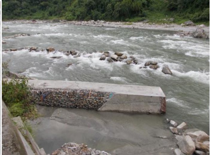
Spurs wall on Sikkim side
